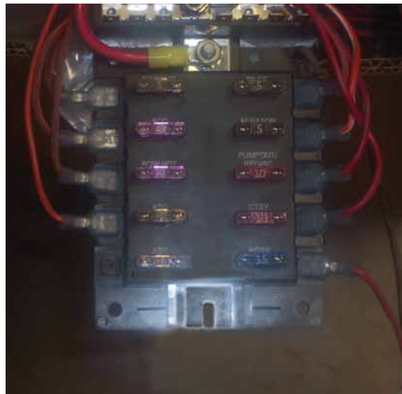
Figure 3-6 SX Fuse Panel
